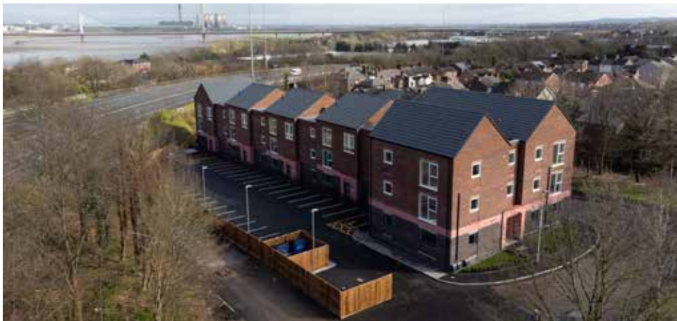
Sewell Street, Runcorn
